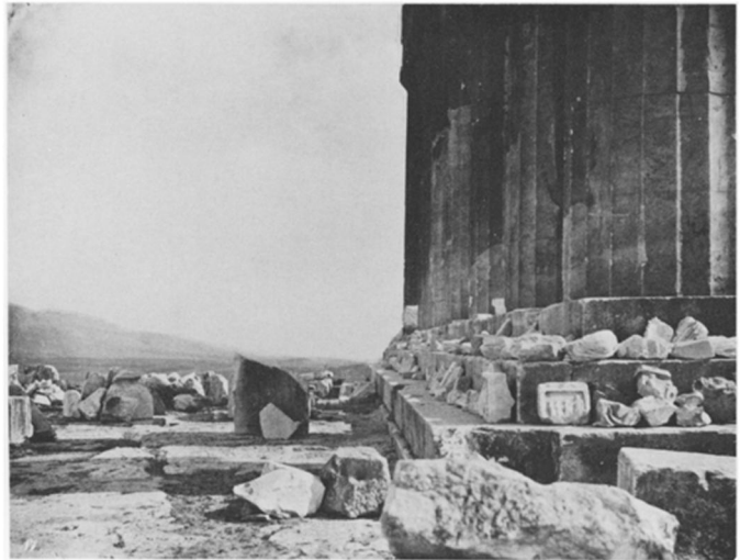
Figure 18. William James Stillman (American, 1828–1901). Profile of the Eastern Facade, Showing the Curvature of the Stylobate , 1869. Carbon print. H: 18.4 cm (7 1 / 4 "); W: 23.7 cm (9 3 / 8 "). Malibu, The J. Paul Getty Museum 84.XO.766.4.18.
